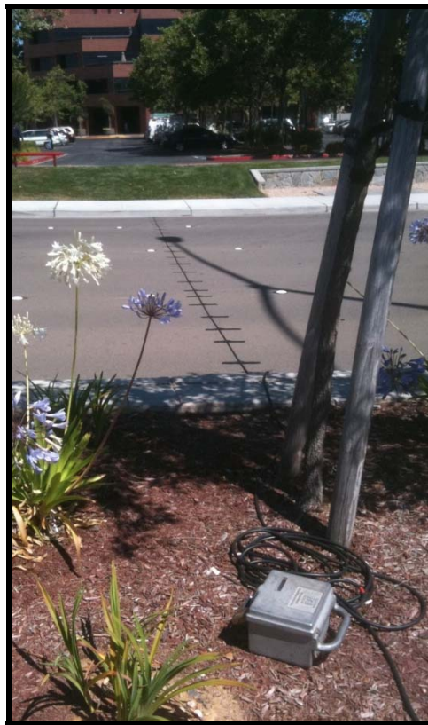
FIGURE 4 ROADWAY TUBE COUNTER HARDWARE
